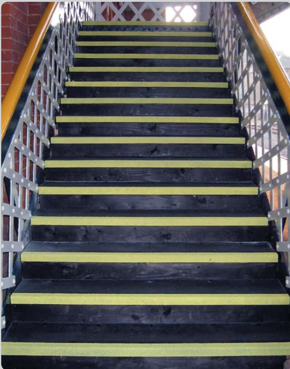
Over-line station bridge
