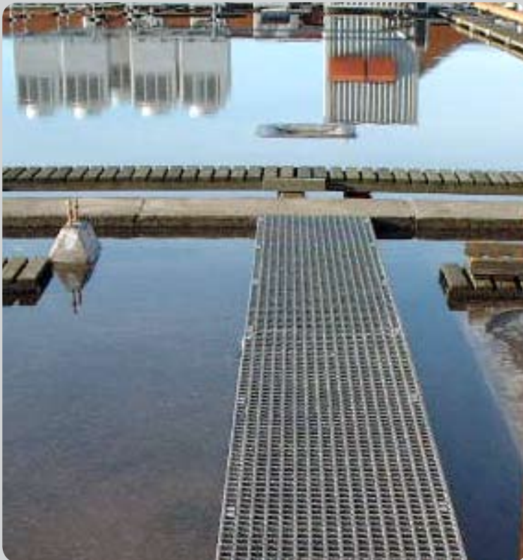
Roof top walkway
